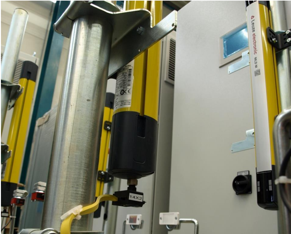
Photo 2. Ready-for-mounting MLD multiple light beam safety devices from Leuze electronic with integrated AS-i interface.
